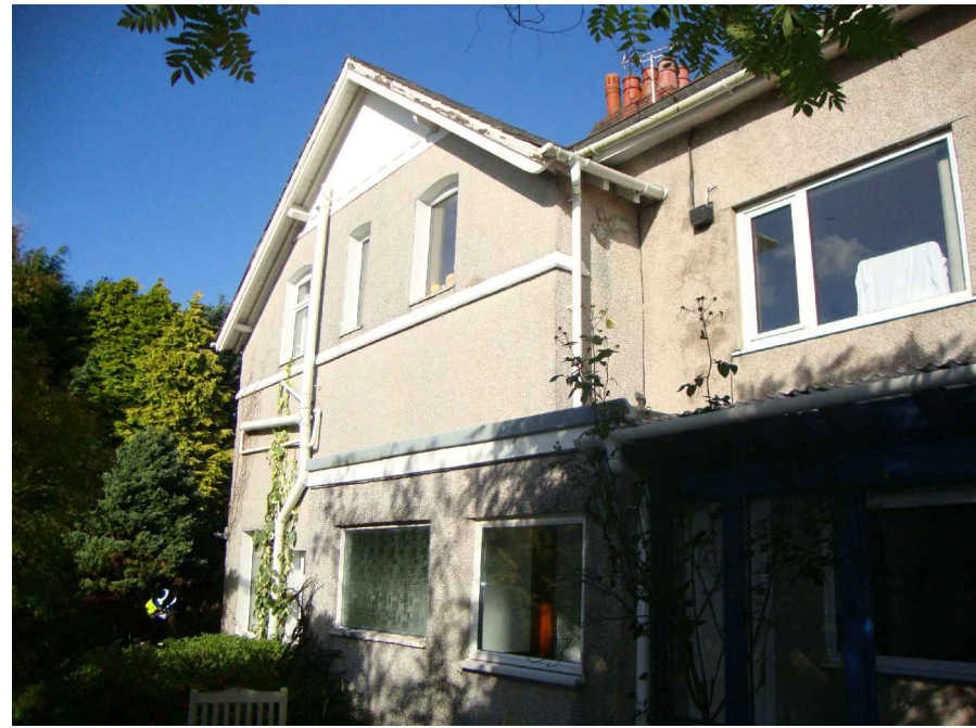
EXISTING SITE PHOTOGRAPHS
